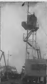
At the start of 1950, new harbor facilities will begin to cut turnaround time even more. This new 75' observation tower; the finished finger pier, and other projects will carry on the job done so well.
